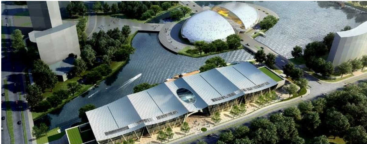
Deqing International Convention Center & Deqing International Exhibition Center
